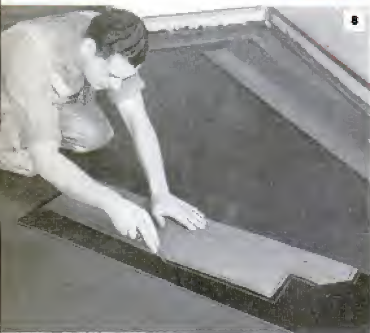
Above, when patterns are used to cut cove, allowance must be made for fitting under cap molding and corners
